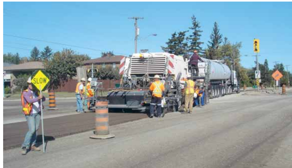
Its engine power of 708 kW provides the 2200 CR with ample reserve capacity for challenging in-situ cold recycling jobs.
